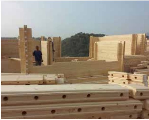
Phase 1 homes made of manufactured logs (3 ply 2x6 SPF).
