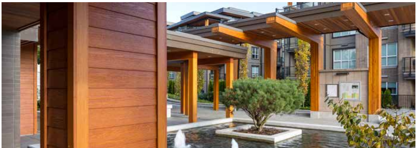
Courtyard of Sail, a six-storey wood-frame construction condo development consisting of 172 units at the University of British Columbia.
