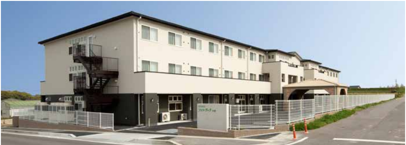
The Flower Search Oobu elderly care facility in Aichi Prefecture, Oobu City, Japan was completed in May 2015. It is a 3,900 m 2 three-story fireproof structure built with SPF dimension lumber.
