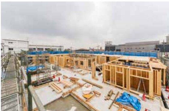
Hanahata Asukaen midply project under construction.
