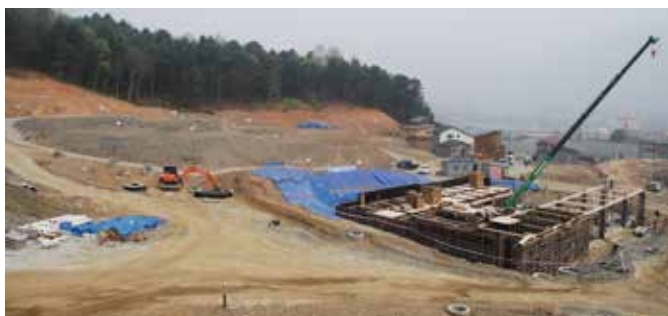
Construction of the project is underway in this May 2014 photo.
