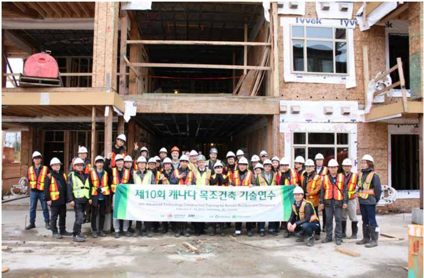
Participants in Canada Wood's Advanced Technology Construction Training program visit a six-storey building under construction in B.C.
