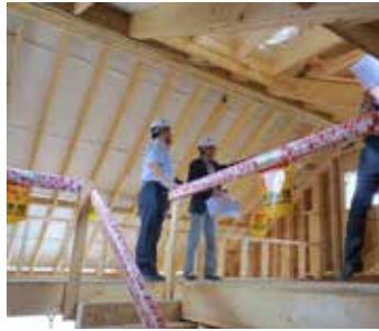
Framing inspection underway at the 5-Star house.
