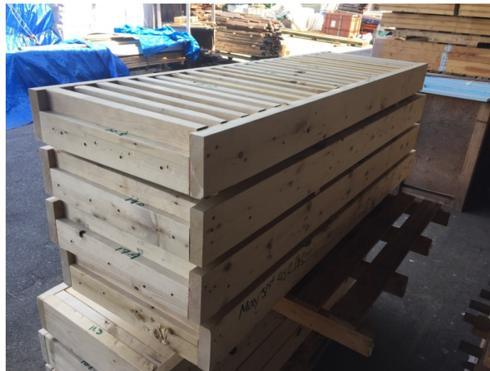
Figure 9. Constructed D panels
