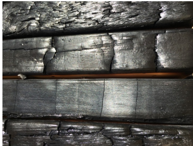
Figure 16. Depth of char between boards in first panel (A assembly)
