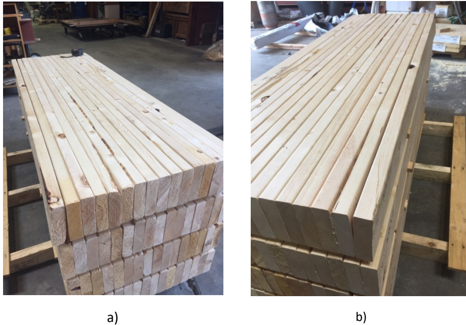
Figure 3. Constructed A panels
