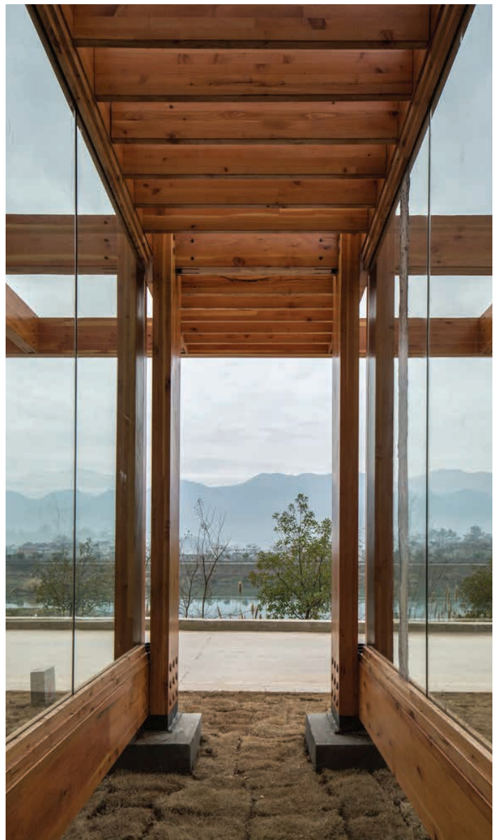
Shimenyu Station, Zhe Jiang.
