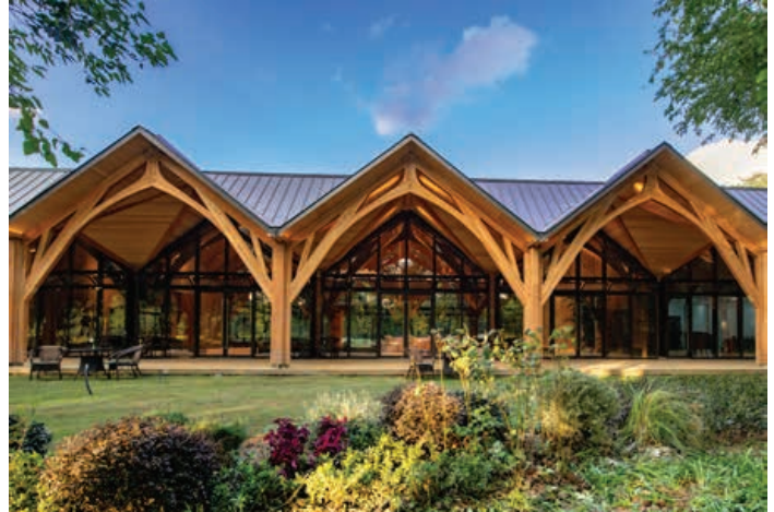
The leaf-shaped roof is supported by glulam beams and the 2x4 purlins create a stunning triangulated structure that weaves sustainable design into the sky. Yi JingYuan Multi-functional Hall, Xijiao State Guest Hotel, Shanghai.
