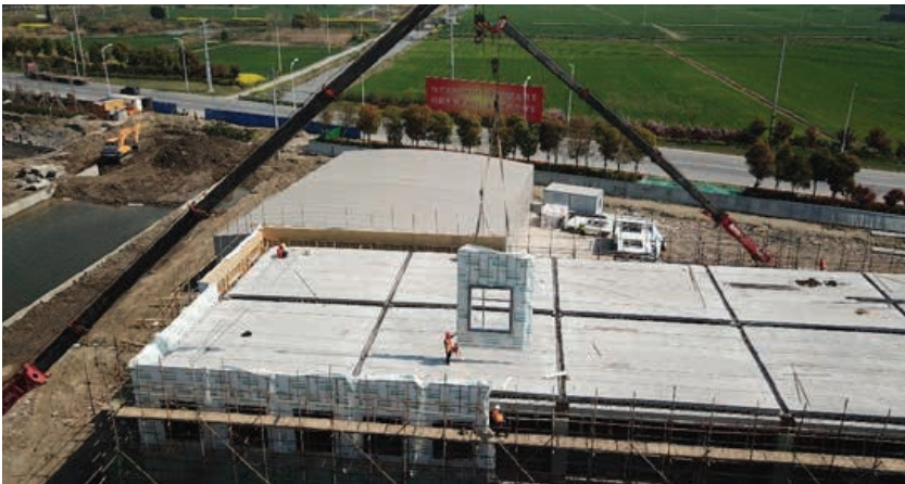
Installation of wood infill walls at the Matechstone Taixing project.
