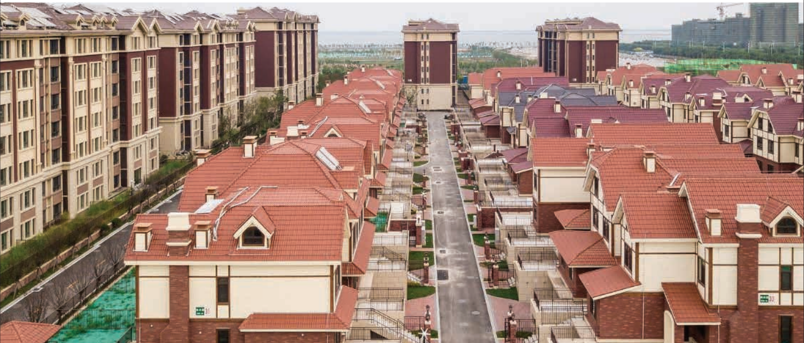
The first phase of the Sino-Canadian eco-district townhouse project, 100 units, was completed in March 2019. These townhouses are part of the Natural Resources Canada led Sino-Canadian Low-Carbon Eco-District in Tianjin. Innovative methods, like infill wood walls and Super-E energy efficiency technologies are used in various parts of the overall project.
