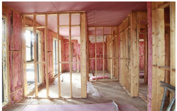
Construction of infill walls of the Jiangsu Yadong Liyang Villa project.
