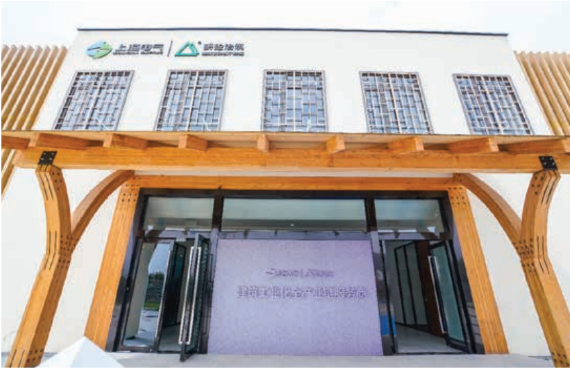
The demonstration Matechstone Taixing project in Jiangsu province, launched in June 2019, is the first commercial project using precast concrete and wood infill wall system in China.
