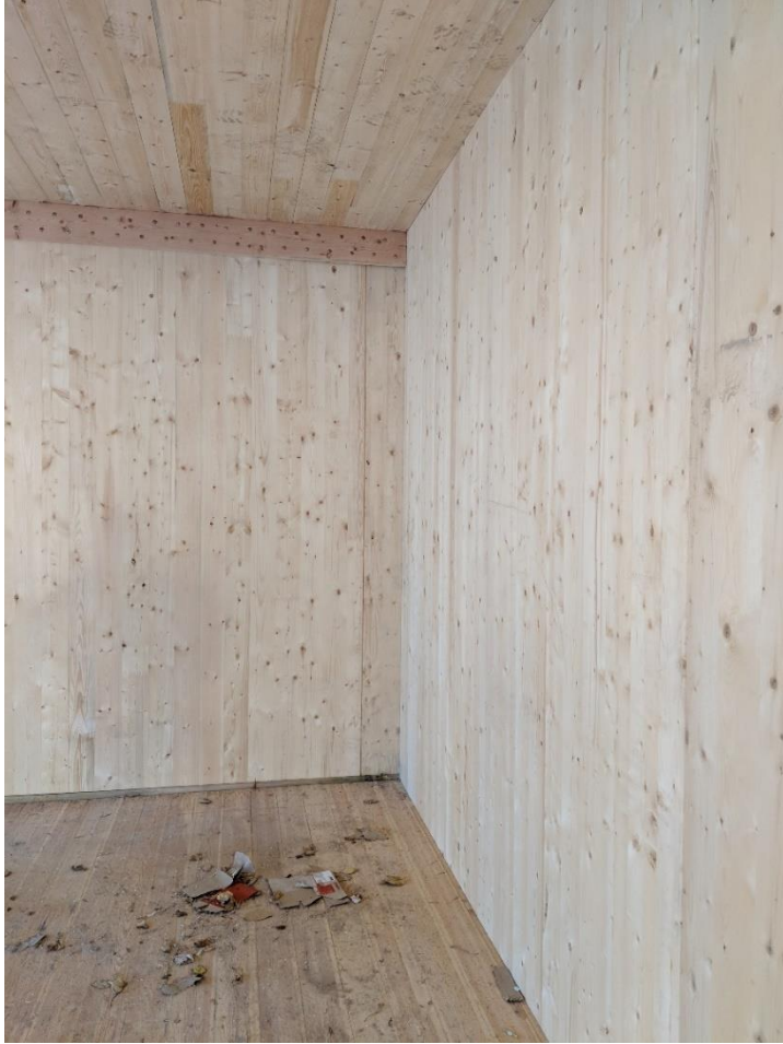
CLT Shear Wall, CREDIT: Fast + Epp
