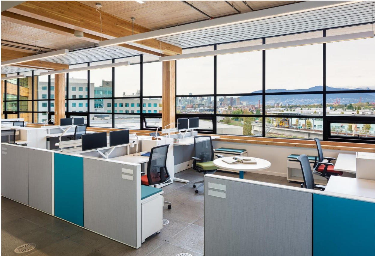
Glulam Post-and-Beam Construction Featured at Mountain Equipment Co-op Head Office, Vancouver, CREDIT: Ed White Photographics
