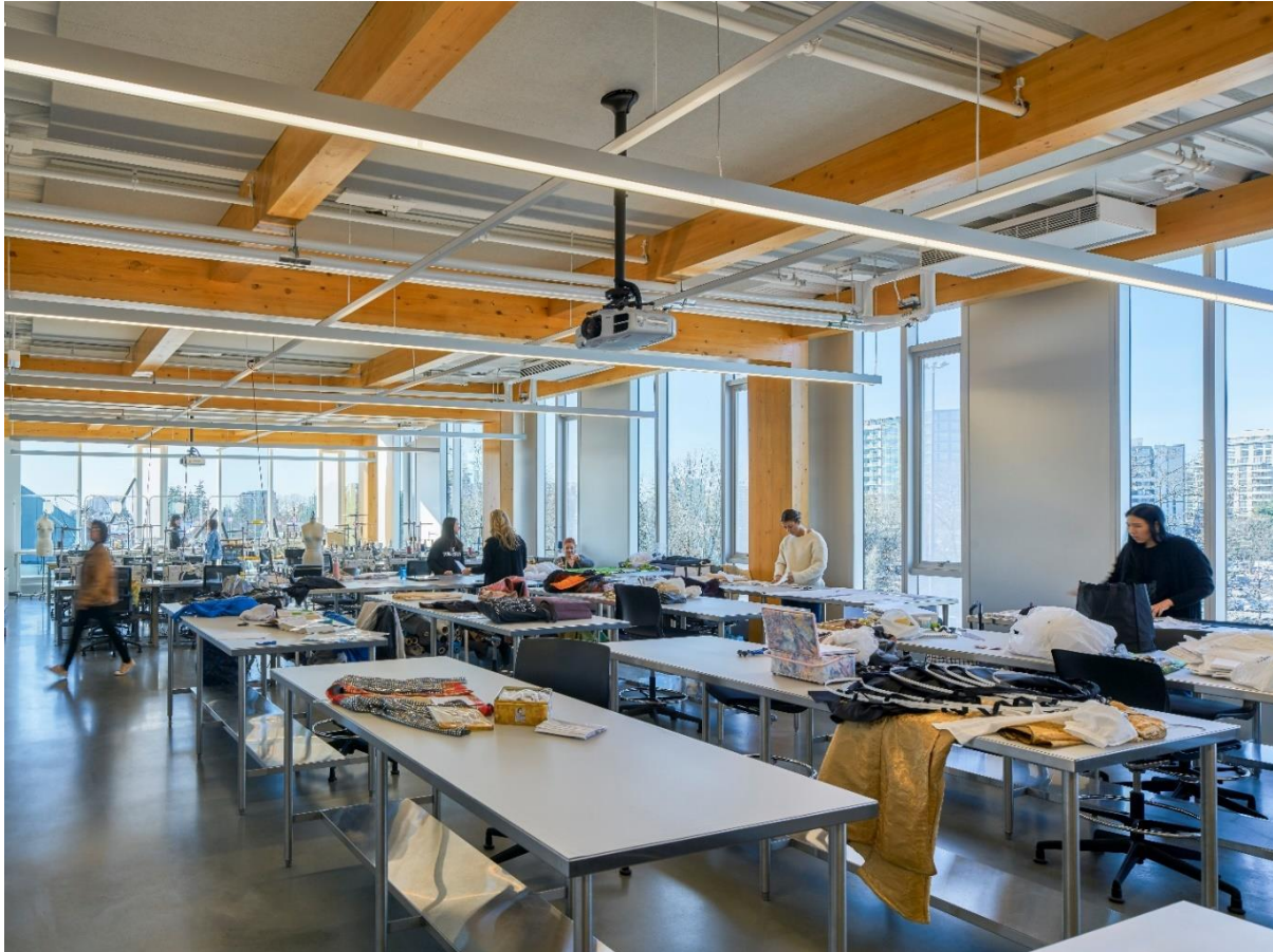
Glulam Post-and-Beam Construction Featured in Wilson School of Design, KPU, Credit: Andrew Latreille Architect: KPMB Architects and Public Architecture + Communication | Engineer: Fast + Epp
