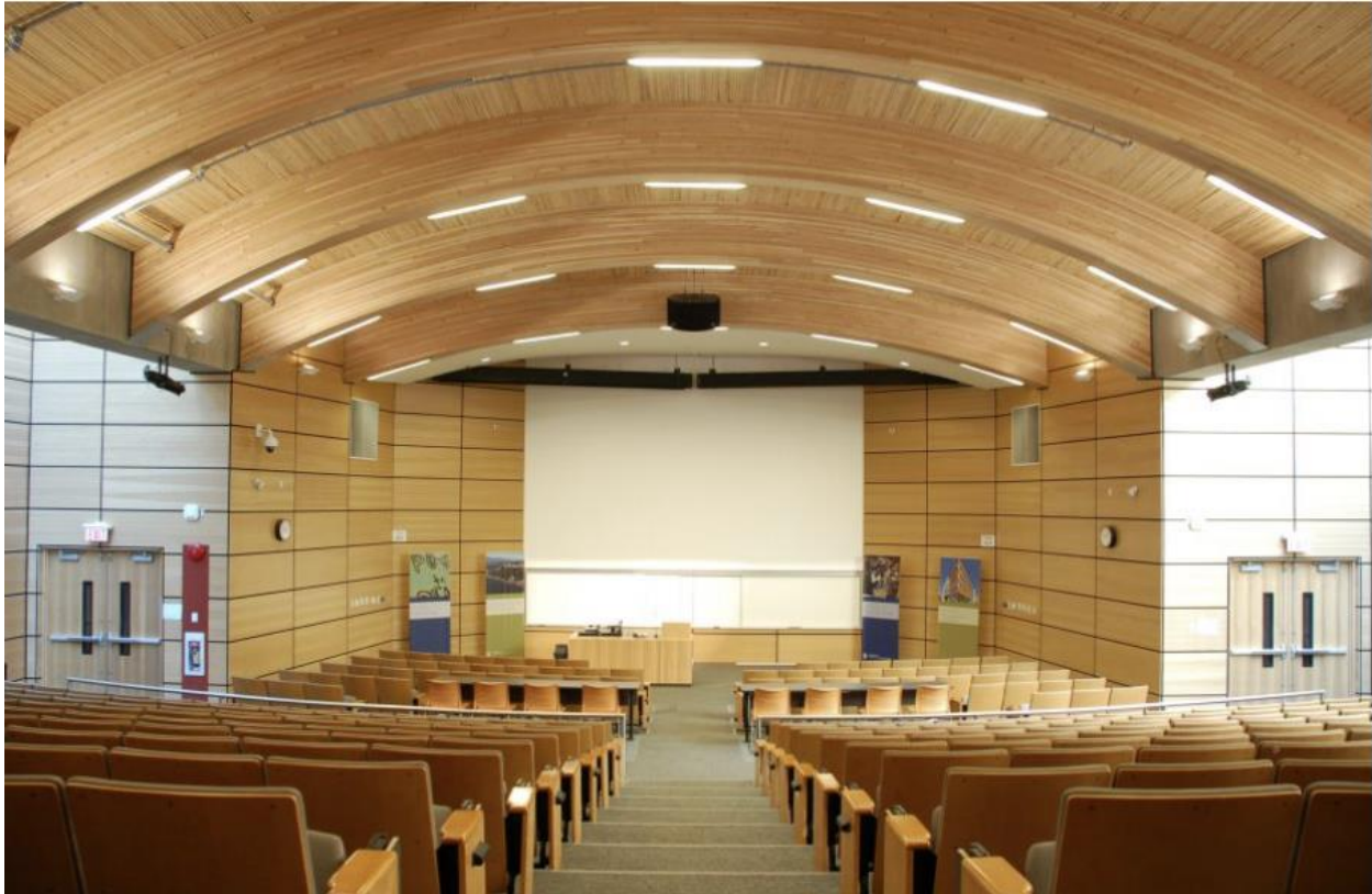
Panel on Purlin Framing Featured at UBC Centre for Interactive Research on Sustainability, CREDIT: Fast + Epp Architect: Perkins + Will | Engineer: Fast + Epp
