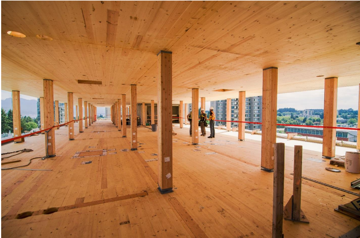
Point-Supported Flat Panel System at Brock Commons, UBC, CREDIT: Neil Taberner Architect: Acton Ostry Architects Inc. | Engineer: Fast + Epp
