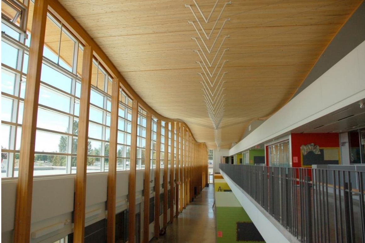
NLT Roof Framing Featured in Samuel Brighthouse Elementary, Richmond BC, CREDIT: Fast + Epp Architect: Perkins + Will | Engineer: Fast + Epp
