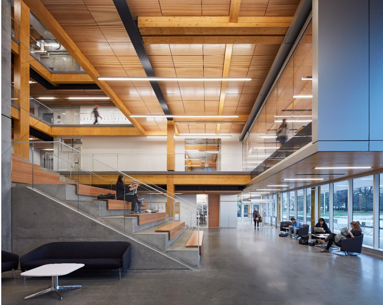
Glulam Post-and-Beam Construction Featured in Wilson School of Design, KPU, Credit: Andrew Latreille Architect: KPMB Architects and Public Architecture + Communication | Engineer: Fast + Epp
