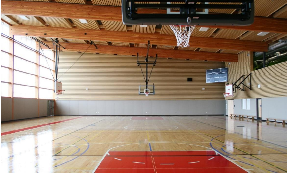
Glulam Post-and-Beam Construction Featured in Richmond Christian School Gymnasium, Richmond BC, Credit: Florian Mauer Architect: Landform Architecture + Design Build | Engineer: Fast + Epp
