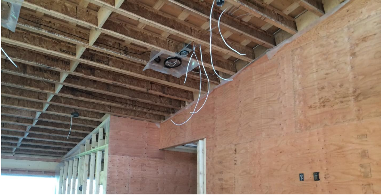
Engineered Lumber Joist Framing, CREDIT: Fast + Epp
