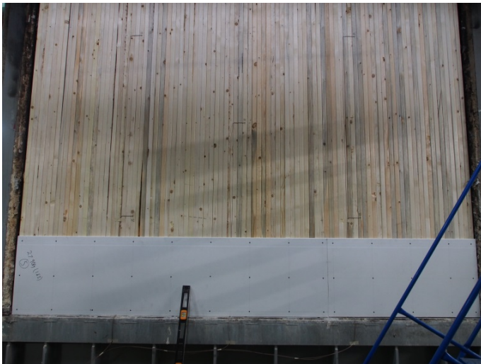
Figure 9. 2x8 NLT wall gypsum installation.
