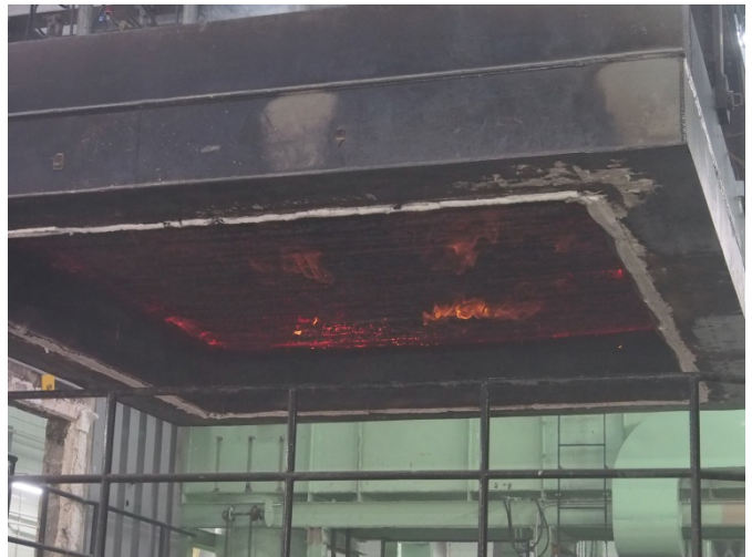
Figure 40. 2x6 NLT floor removal from furnace.
