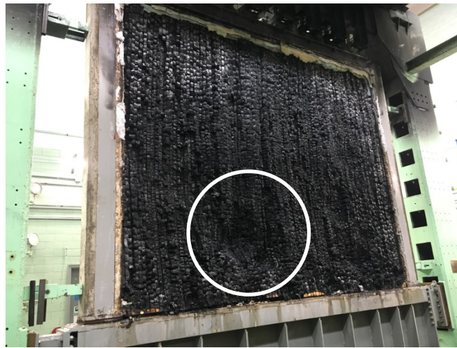
Figure 32. 2x8 NLT wall exposed surface after test, depression.
