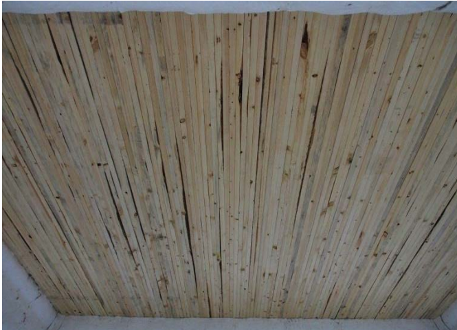
Figure 15. 2x6 NLT floor, exposed surface.
