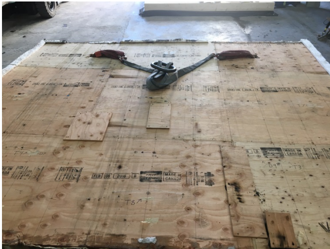
Figure 26. 2x6 NLT wall layout of added plywood pieces.
