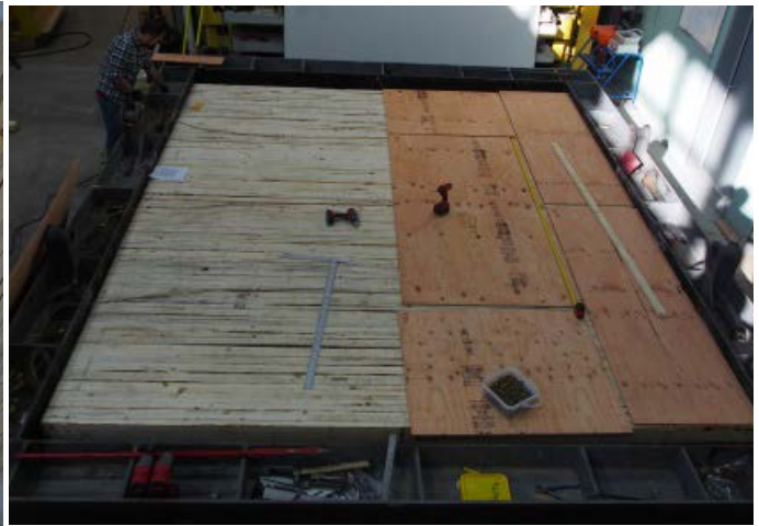
Figure 16. 2x6 NLT floor, installation of plywood.
