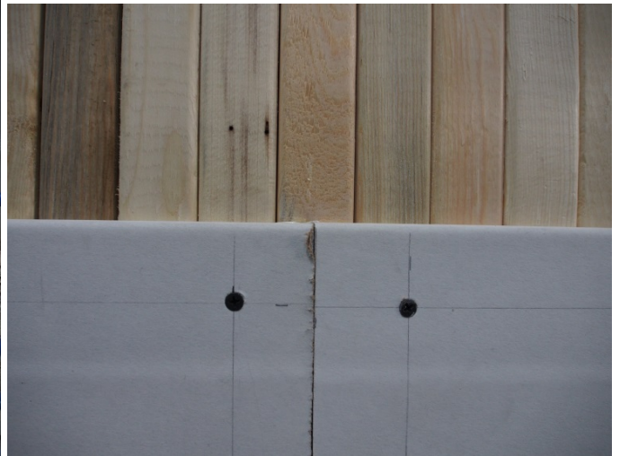
Figure 10. 2x8 NLT wall gypsum joint alignment.
