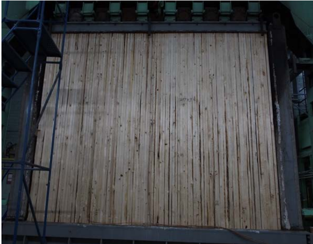
Figure 2. 2x6 NLT Unexposed side before plywood installation.
