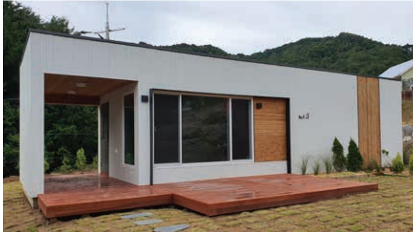
Photos: Smart House, Haruhome
