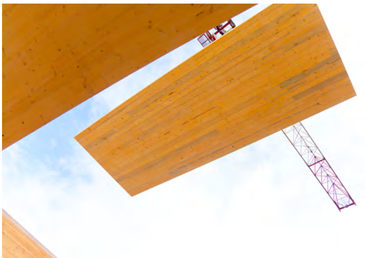
Cross-laminated timber installed during construction of the Earth Sciences Building at the University of British Columbia | Photo: KK Law
