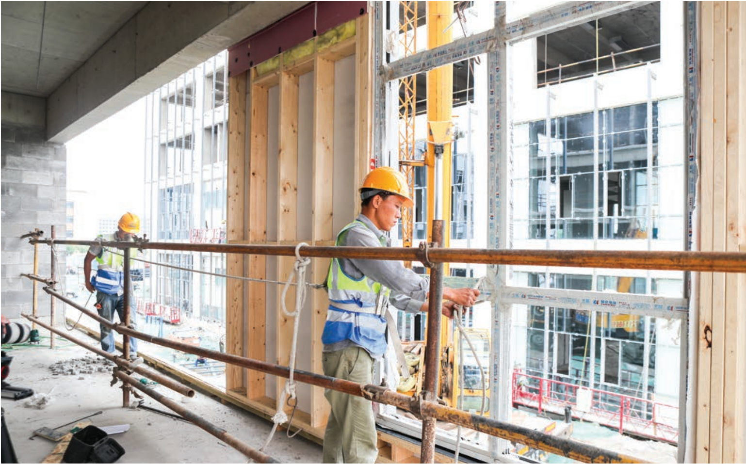
C-Mars Office Project—installing the prefabricated wood wall | Photo: Canada Wood China
